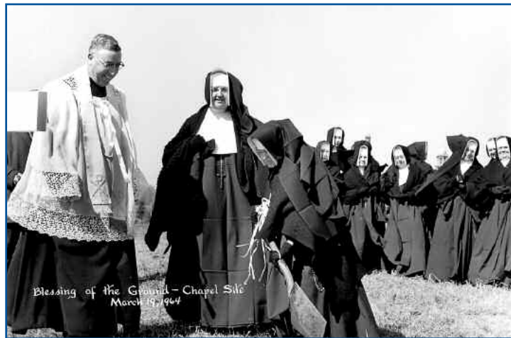
Father Hugh Nolan, Mother Maria Pacis, Mother Maria Alma breaking ground for the new Motherhouse at Immaculata, March, 1964
